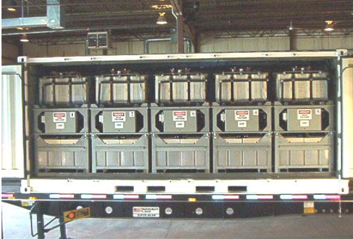
Figure 2. A 250-kWh string of five modules in a standard shipping container.
